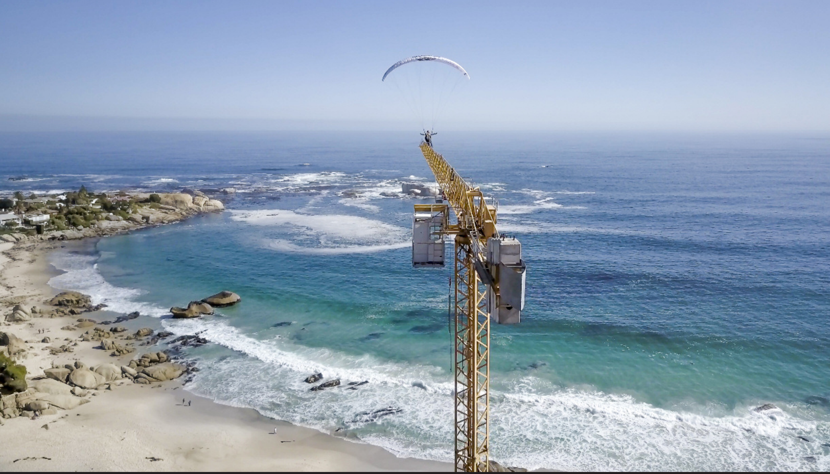
According to JBC, the crane was the most difficult obstacle. It isn't obvious how to assess distances in 3D with metal tubes.
